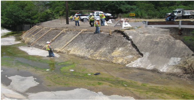
Concrete Rip Rap Channel Wall Repair (Sealing Channel)
