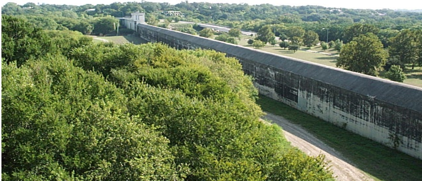
Olmos Dam After Retrofitting
