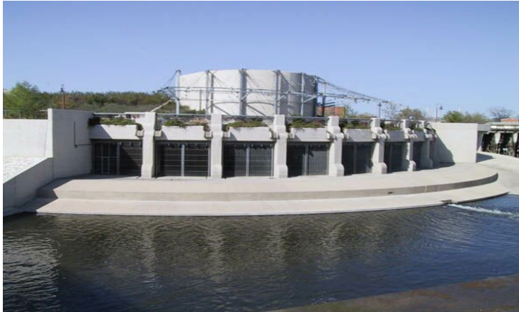
San Antonio River Tunnel Outlet
